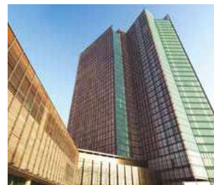
Al Maryah Island Four Seasons Hotel Abu Dhabi, United Arab Emirates
